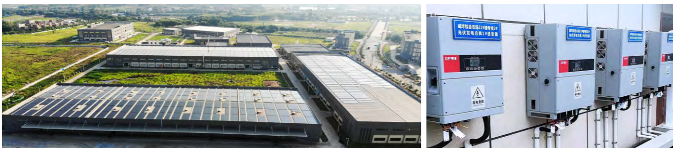
4.557MW p Inverters: 90* Suntrio Plus 40K/50K Address: Qingyuan Guangdong
